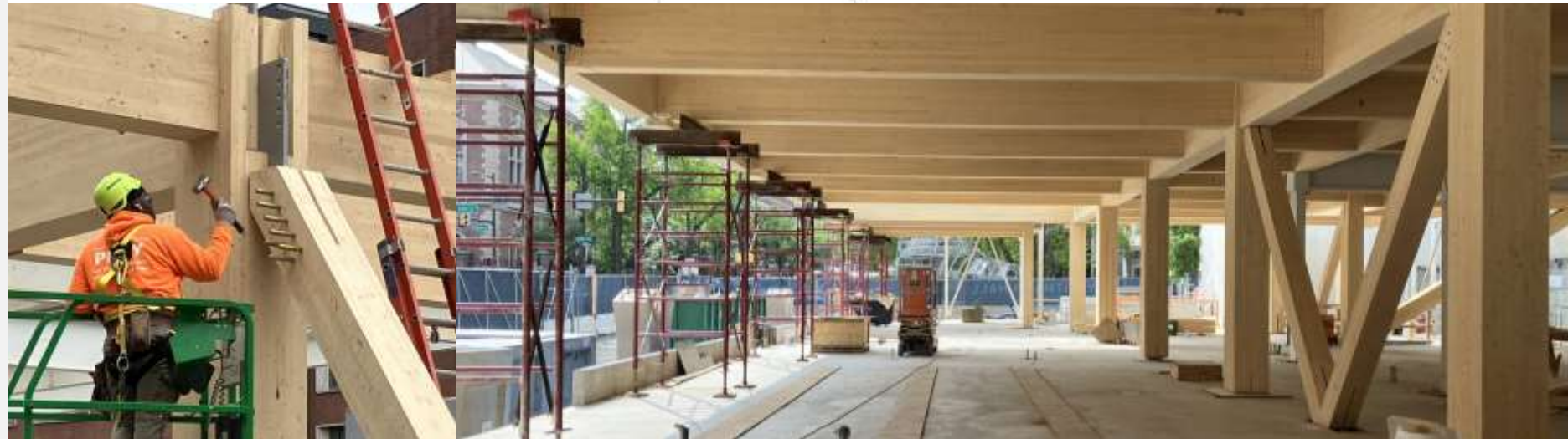
TYPICAL GLULAM BEAM TO COLUMN SHEAR CONNECTION
