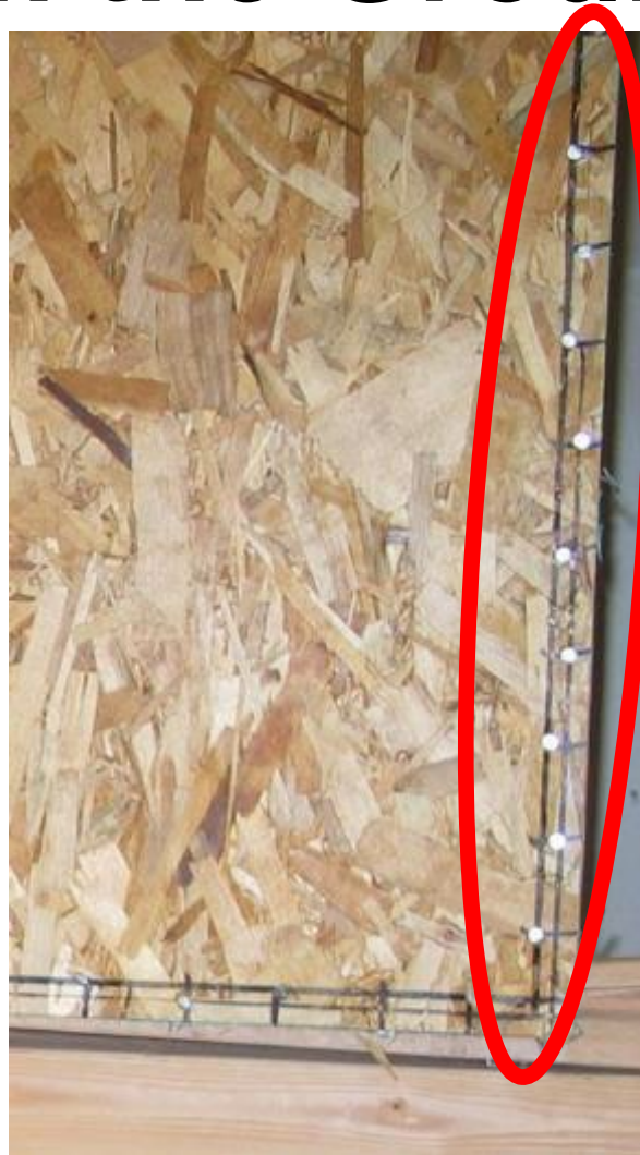
Nailing not staggered
