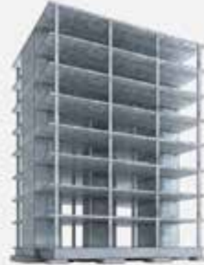
Reference 2 Concrete Flat Slab; Concrete Cores
