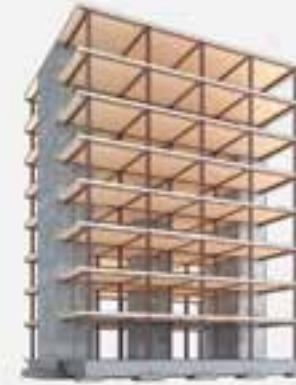
Timber Use 1 Timber Floors; Steel Frame; Concrete Cores
