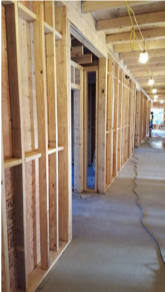
Light Wood-Frame Photo: WoodWorks
