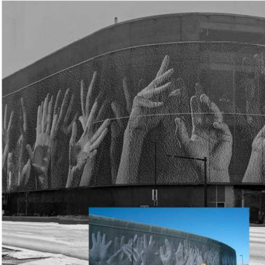
Commissioned artist Christian Moeller photographed hands of various San Jose residents for San Jose Airport garage
