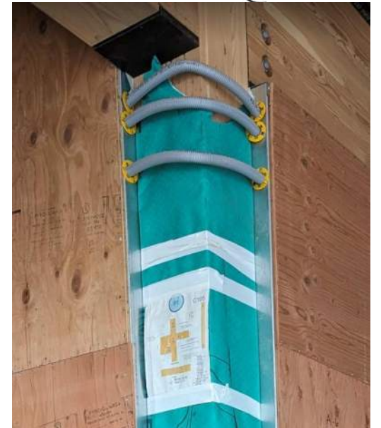
TYPICAL CROSS-LAMINATED TIMBER PANEL EDGE AT SHEAR WALL
