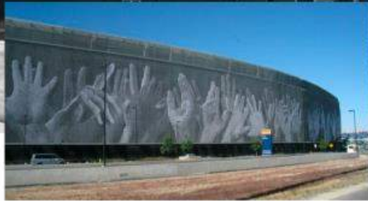
Custom pucks snapped on chain link mesh, 1200' long, 7 stories high
