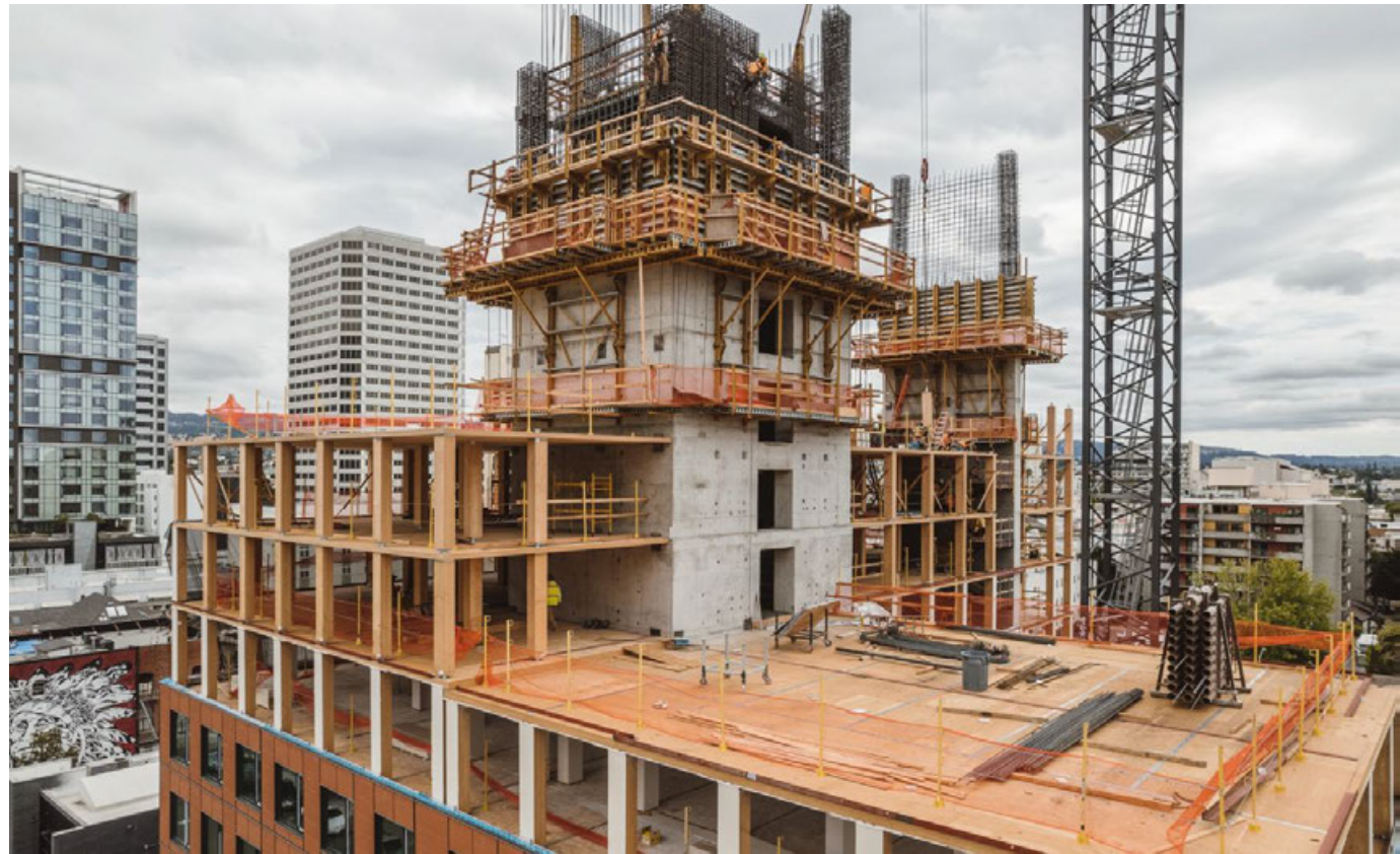
1510 Webster / oWow / DCI Engineers / Photo Flor Projects
