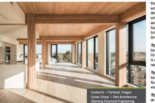
A building's assigned construction type is the main indicator of where and when all wood systems can be used. IBC Section 602 defines five main options (Type I through V) with all but Type IV having subcategories A and B. Types III and V permit the use of wood framing throughout much of the structure and both are used extensively for modern mass timber buildings.
