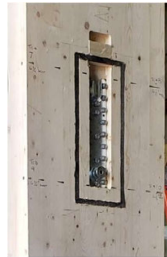
Intumescent fire seal to column prior to beam installation
