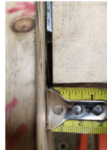
Gap between glulam beam end and glulam column face after installation
