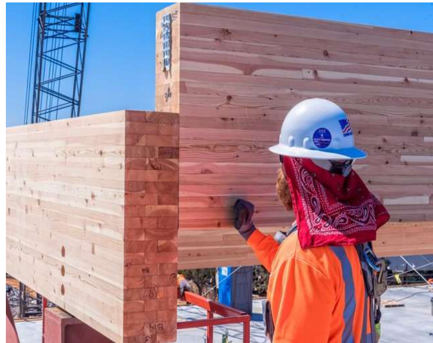
Assembly of glulam beam to column connection (image: DPR Construction)
