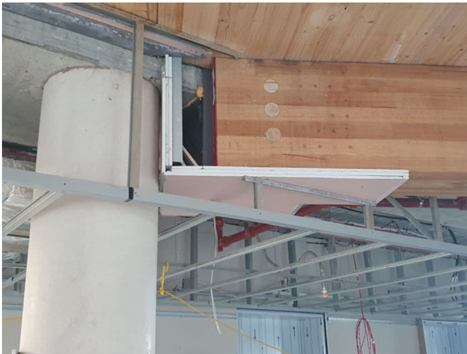
External steel plate connectors in the process of being protected by fire rated gypsum board
