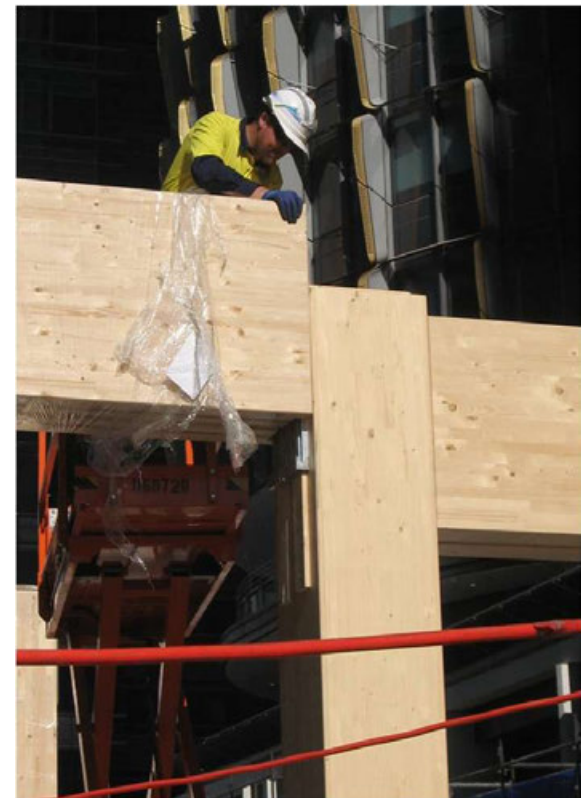
Concealed metallic connectors – site assembly
