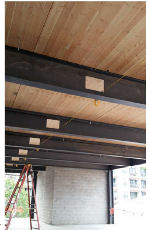
Steel beams protected with intumescent paint supporting CLT floor
