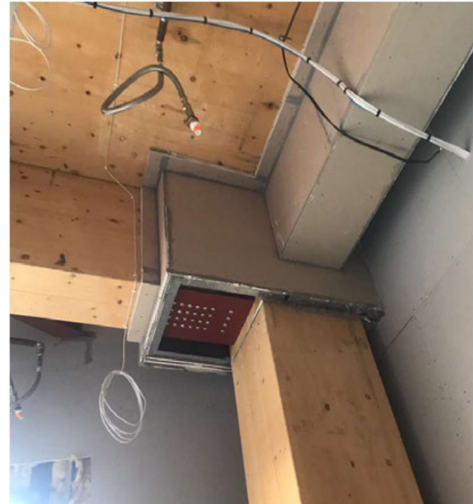
External steel plate connectors in the process of being protected by fire rated gypsum board
