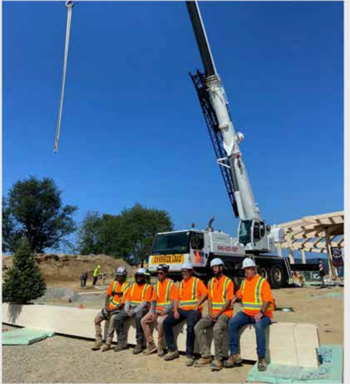
Photo : Consigli Construction
