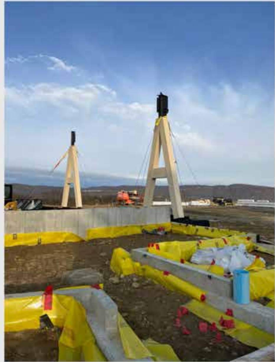
Photo : Consigli Construction
