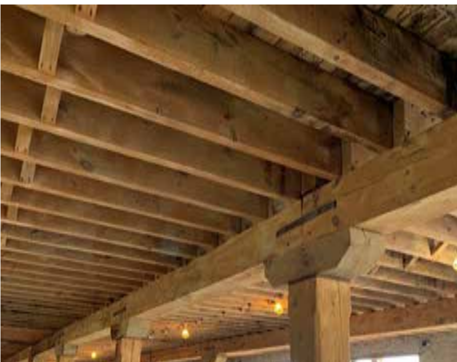
EXISTING FLOOR/CEILING ASSEMBLY
