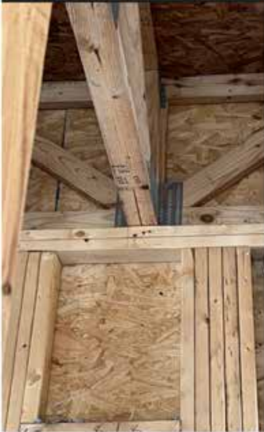
misaligned bearing studs | alternate details
