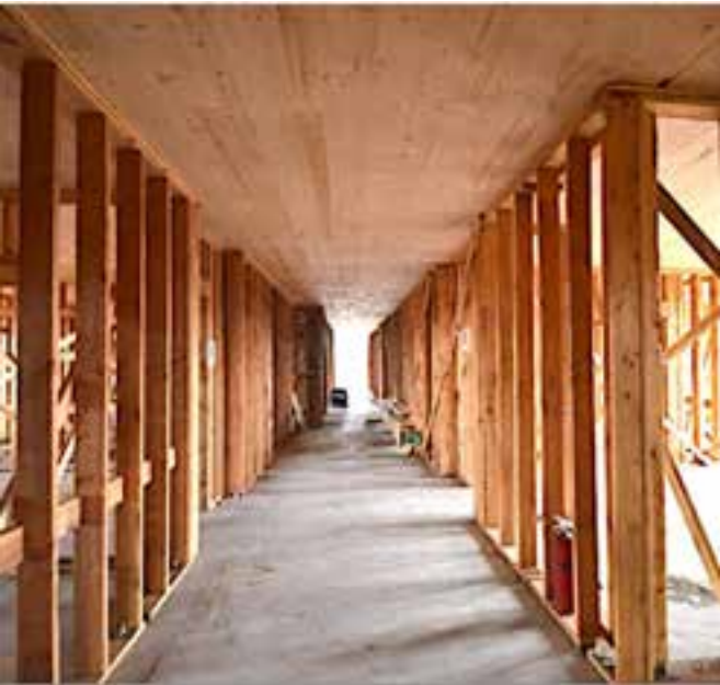
MT Floors & Roofs on LWF Bearing Walls
