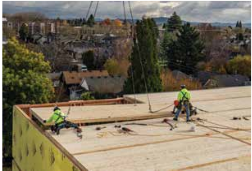
Panel to Support w/ Screws
