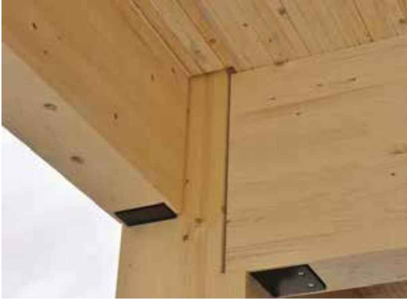
Partially Concealed Connectors
