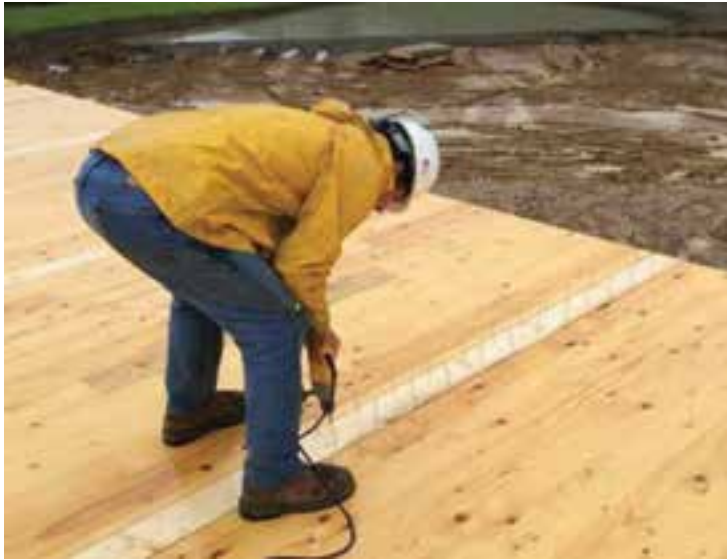
Panel to Panel Spline w/ Screws
