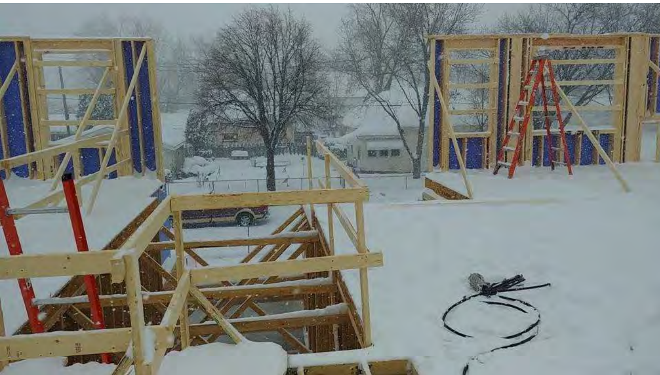
Standard: Platform Framing
