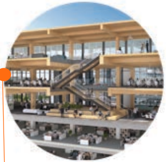
80 M Street Washington DC 10 stories – 3-story mass timber vertical addition
