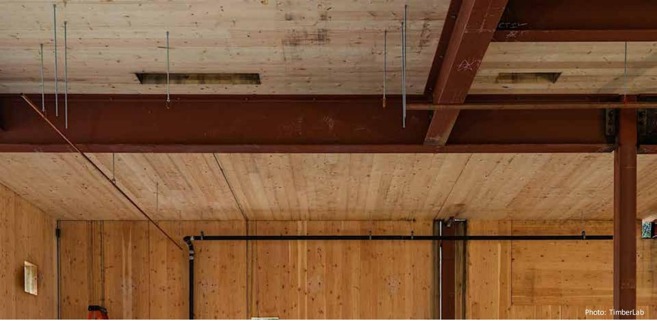
**STRUCTURAL SOLUTIONS** | HYBRID STEEL + MASS TIMBER
