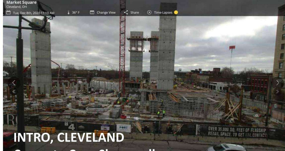
**Concrete Core Shearwalls**
