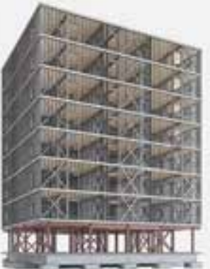
Timber Use 3 Timber Floors; LGM Framing; Steel Frame Podium
