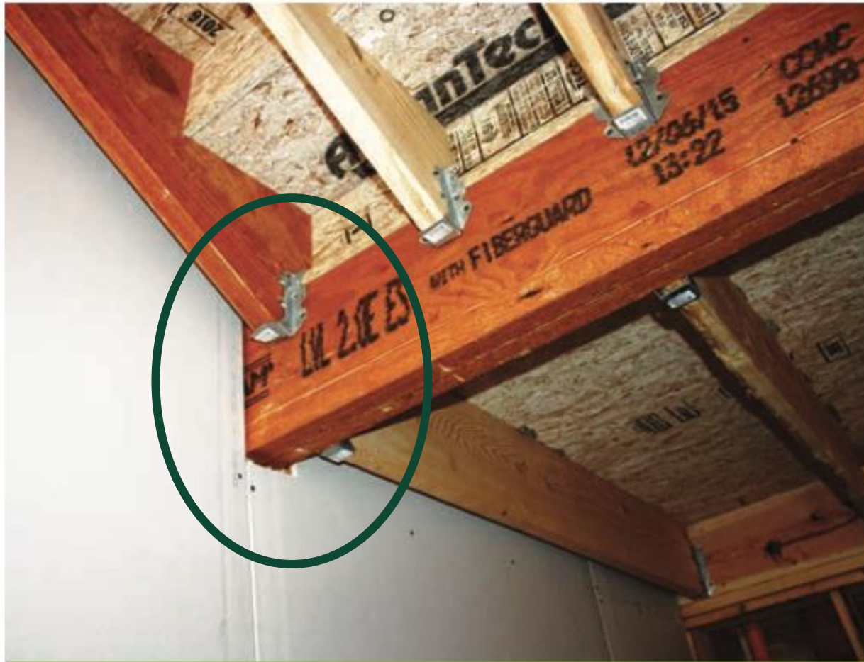
Stair landing beam shaft wall structural penetration prior to firestop system installation
