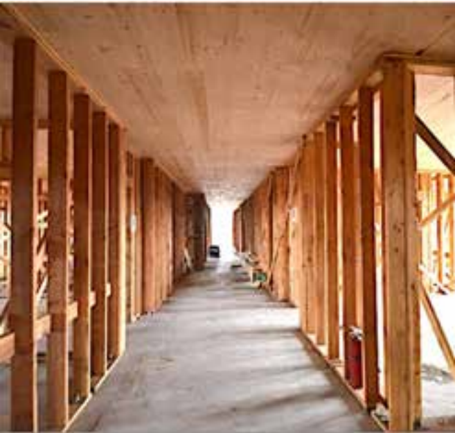
MT Floors & Roofs on LWF Bearing Walls
