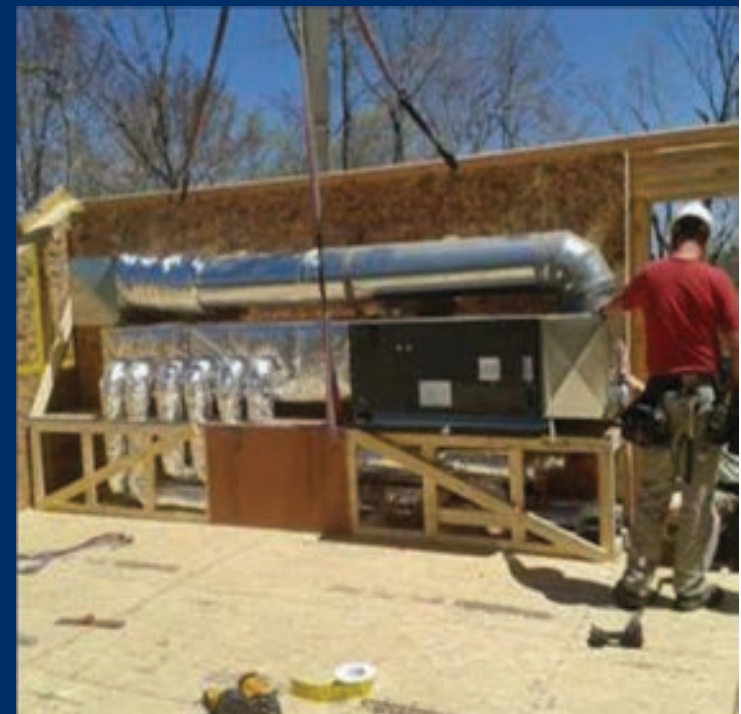
Cartridge Installation
