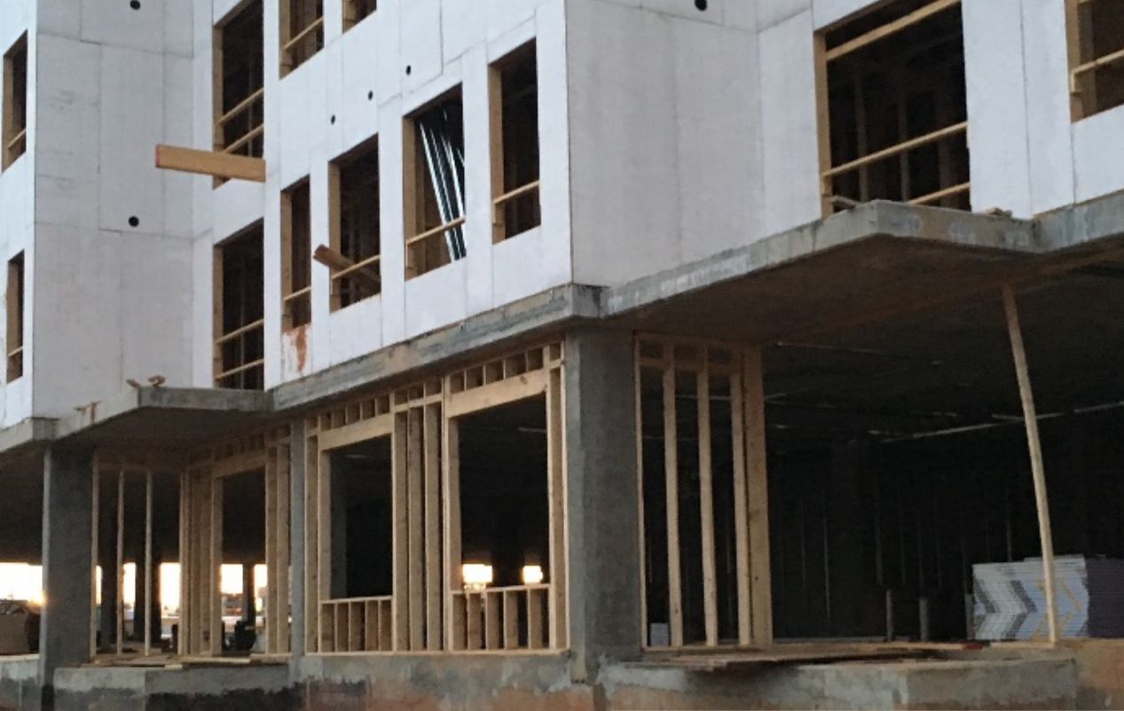
2X6 WOOD STUDS W/ R-21 BATT INSULATION
