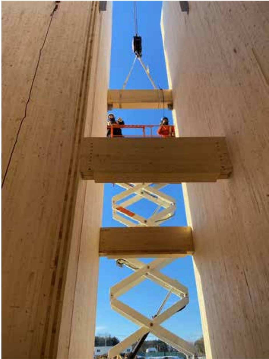
CLT Shear Walls
