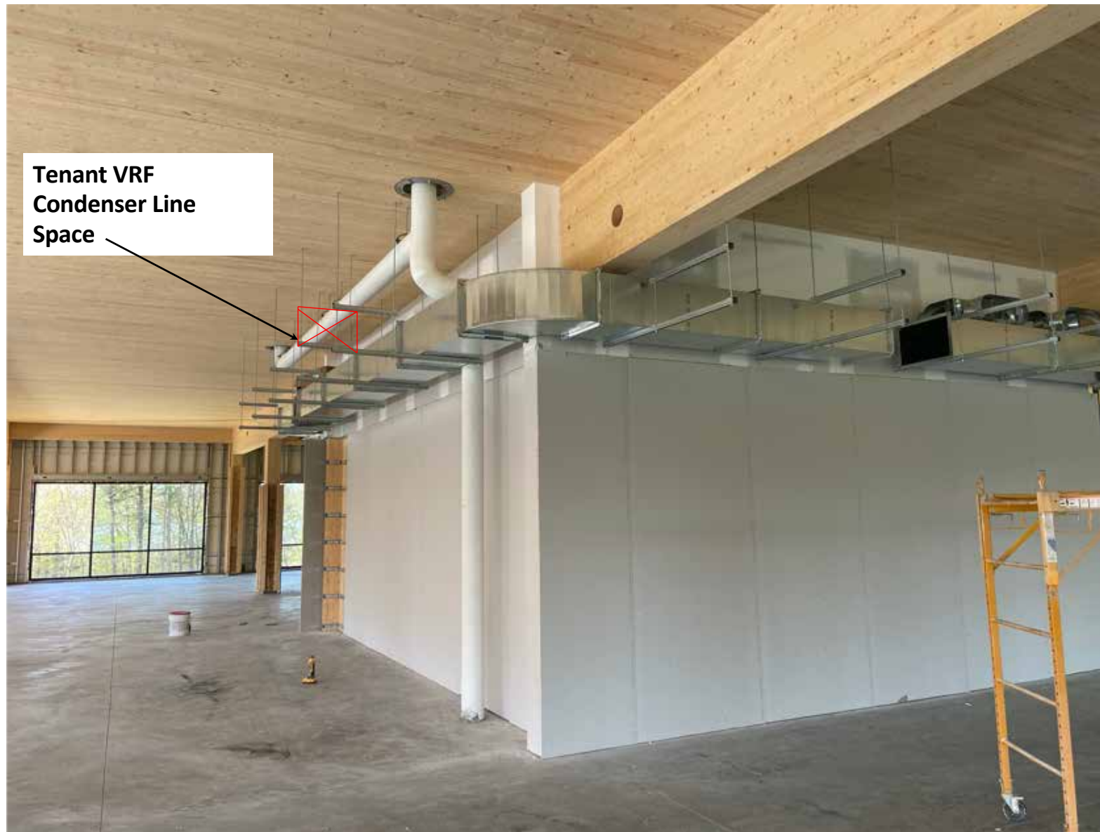
HVAC System Under Construction
