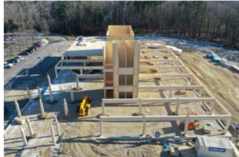
90 Arboretum CLT Shear Wall Core & Framing
