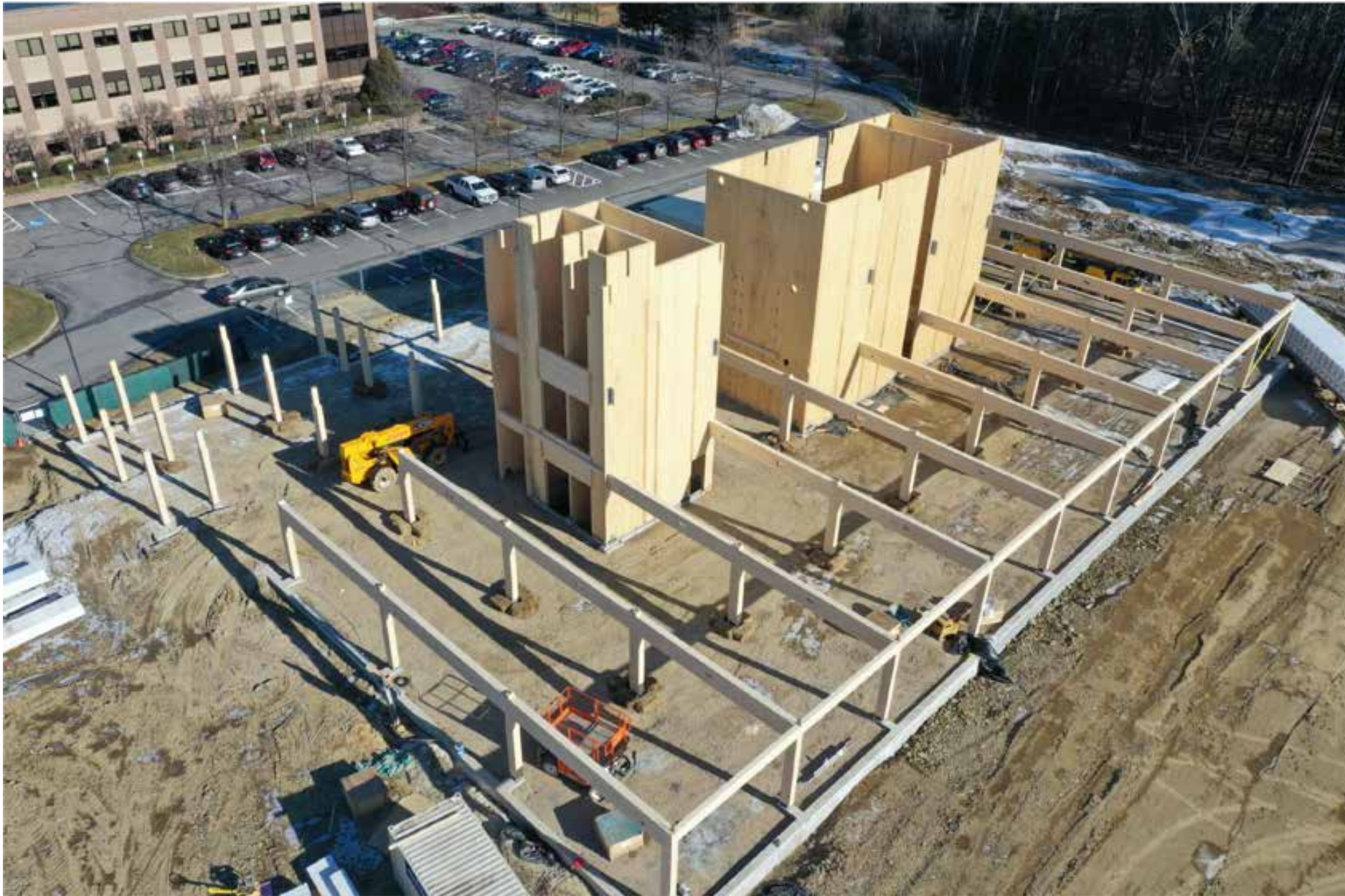
CLT Shear Walls + Framing
