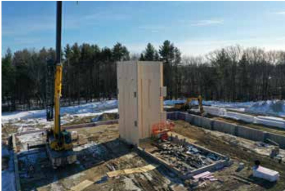
90 Arboretum CLT Shear Wall Core
