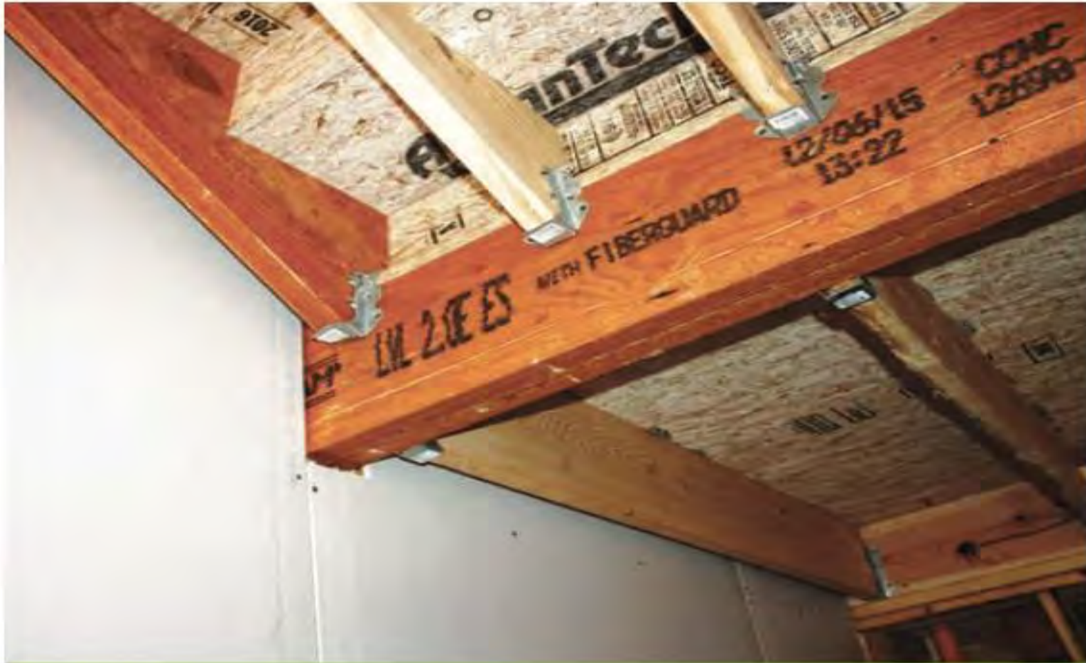
Stair landing beam shaft wall structural penetration prior to firestop system installation
