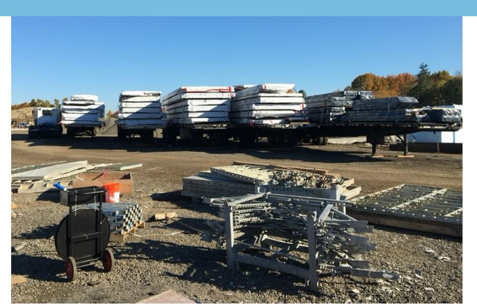
Logistics, laydown space, truck flow is critical to speed of installation.
