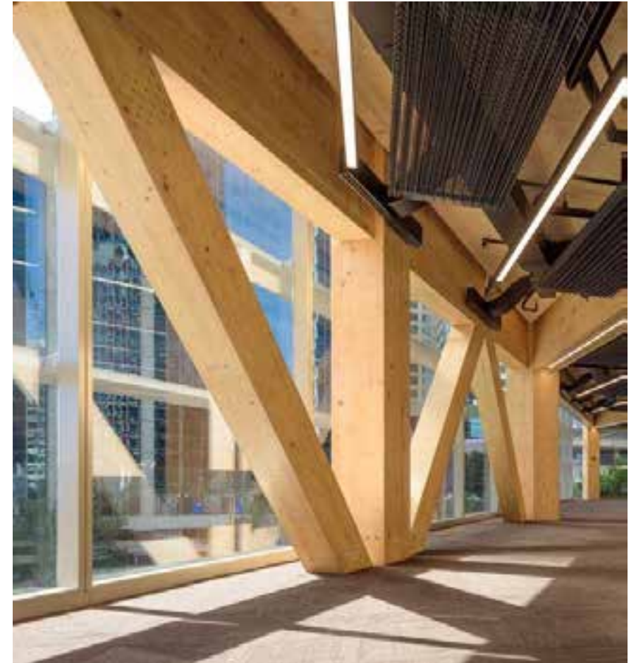
International House, Sydney | Image Credit: HESS
