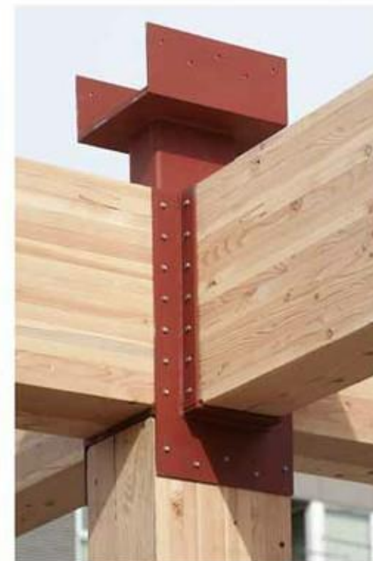
Glulam column caps at the Bullitt Center
