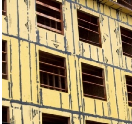
Sealed Gypsum Sheathing – Sealant Filler at Joints
