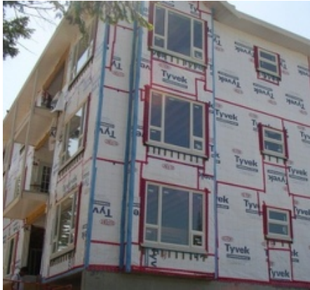
Loose Sheet Applied Membrane – Taped Joints & Strapping
