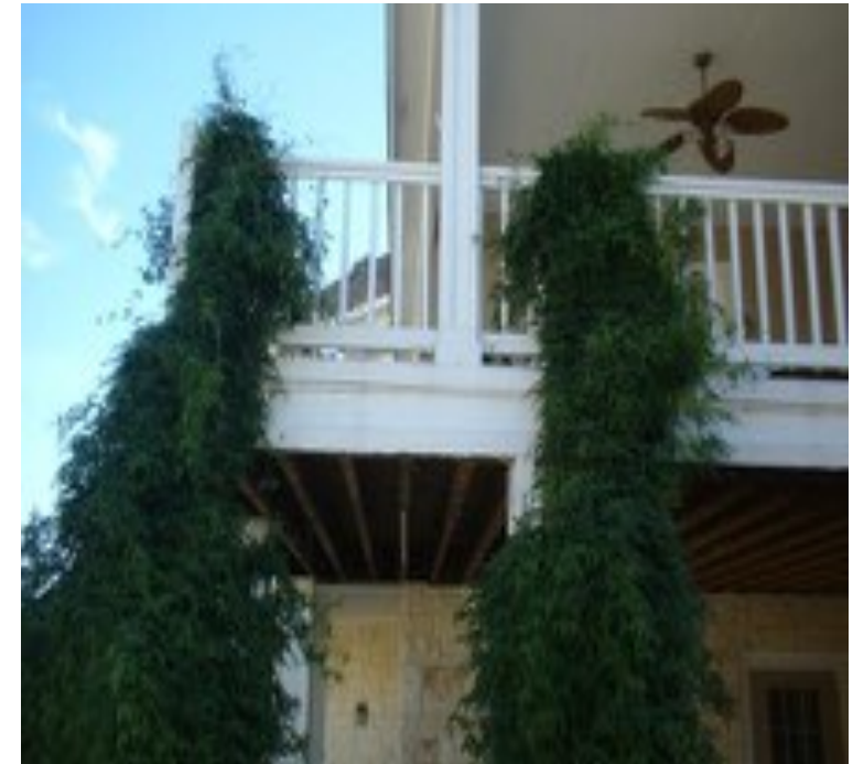
Townhome Open Balcony Framing Partial Roof Protection?
