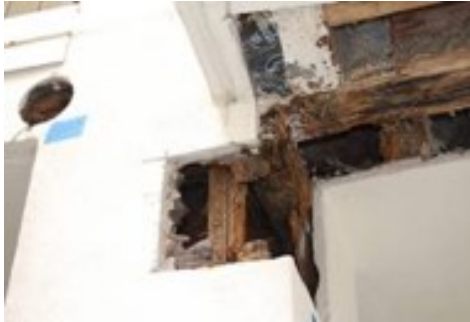
Condos – La Jolla, CA Balcony Framing Moisture Intrusion into the Building Envelop
