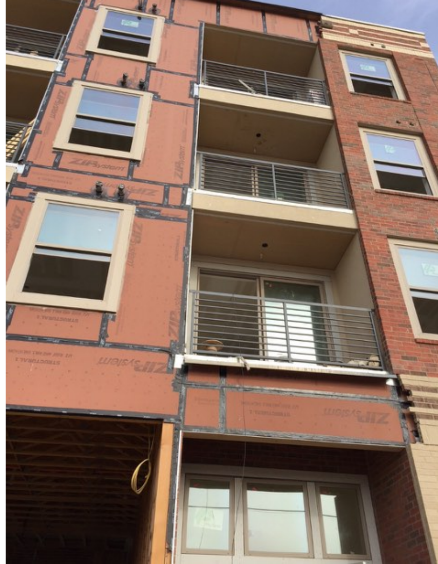
HDH Complex – Frisco, TX Waterproof Membrane Perforated Vinyl
