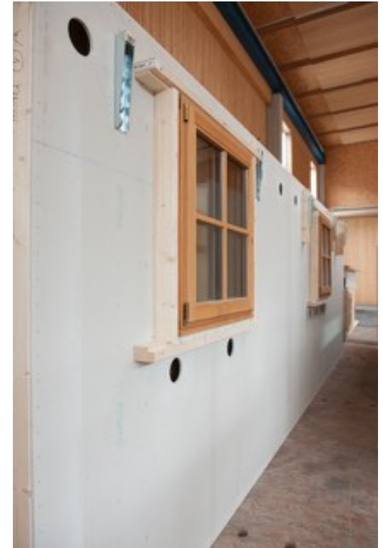
Layer attaching to exterior wall
