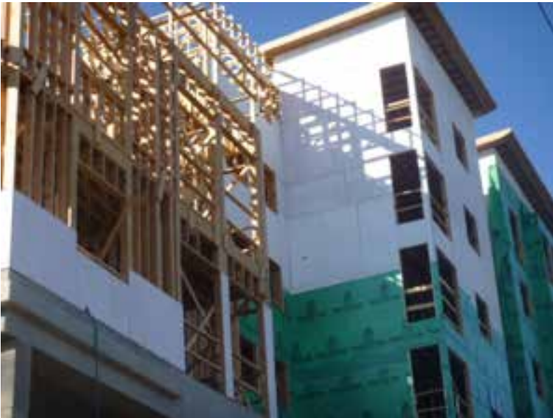
2-hour rated wall assembly with FRCC OSB in Type III construction (Student housing, College Park, MD)
