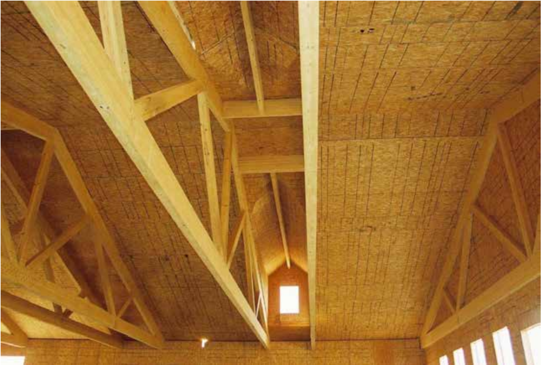
90ft Span Concealed Connector Timber Truss
