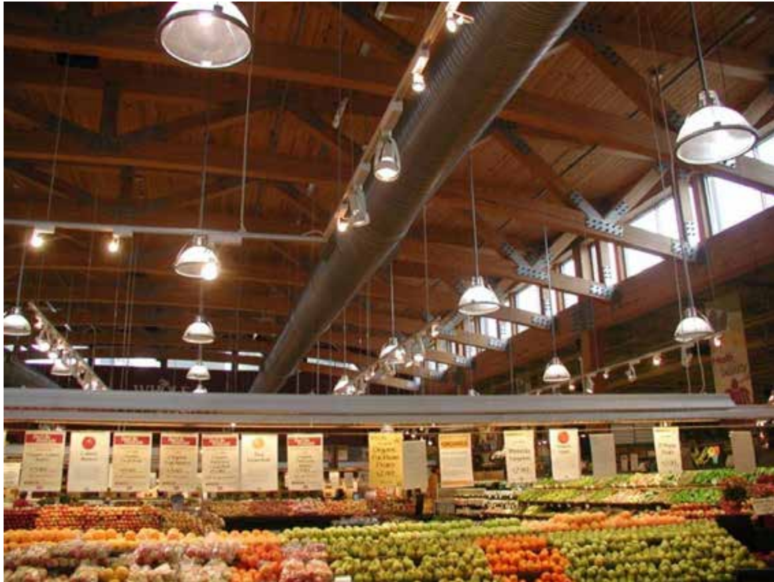
67' Span Glulam Trusses
