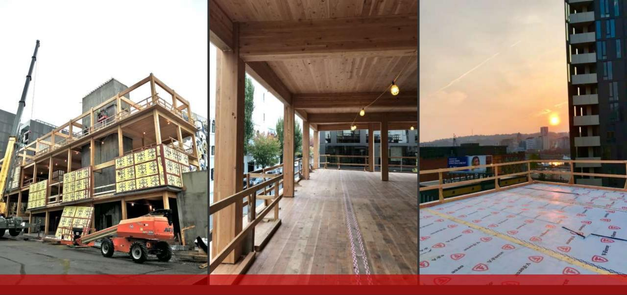
Working the plan: Prefabricated Wall Elements, shop installed roof vapor barrier.
