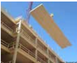
Nail-Laminated Timber (NLT)
