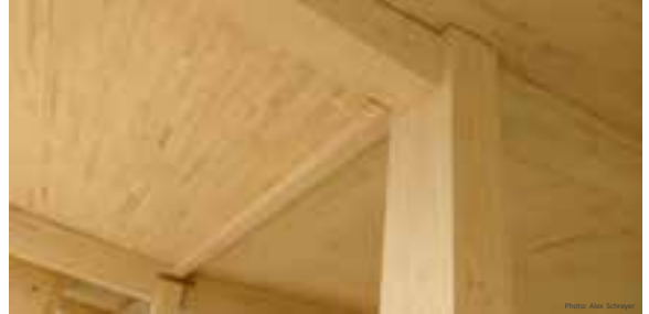
Glue Laminated Timber (GLT)
