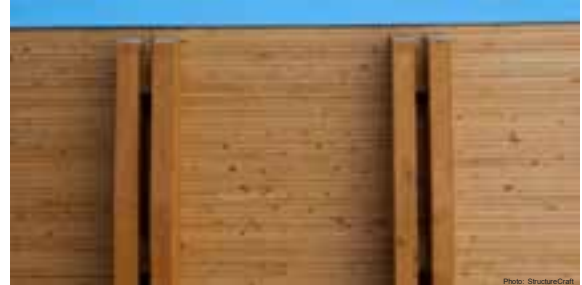
Nail-Laminated Timber (NLT)
