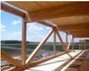
Glue Laminated Timber (GLT)
