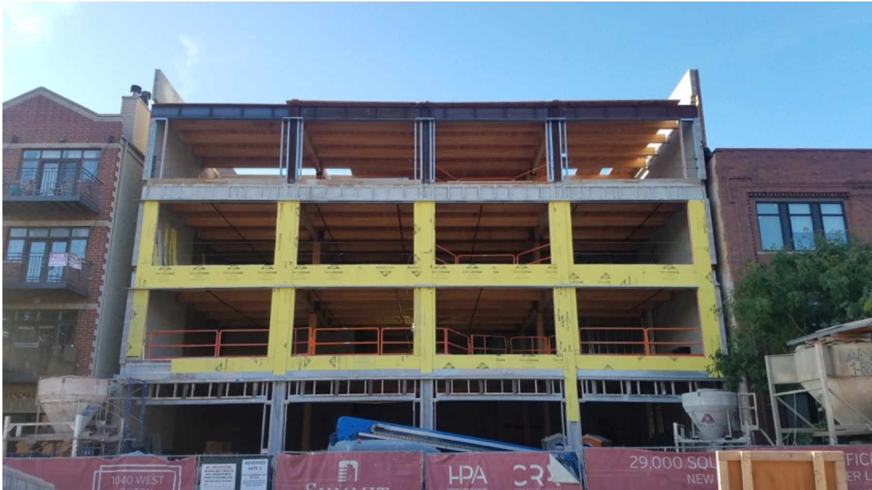
EXTERIOR FRAMING AND AWB INSTALLATION IN PROGRESS
