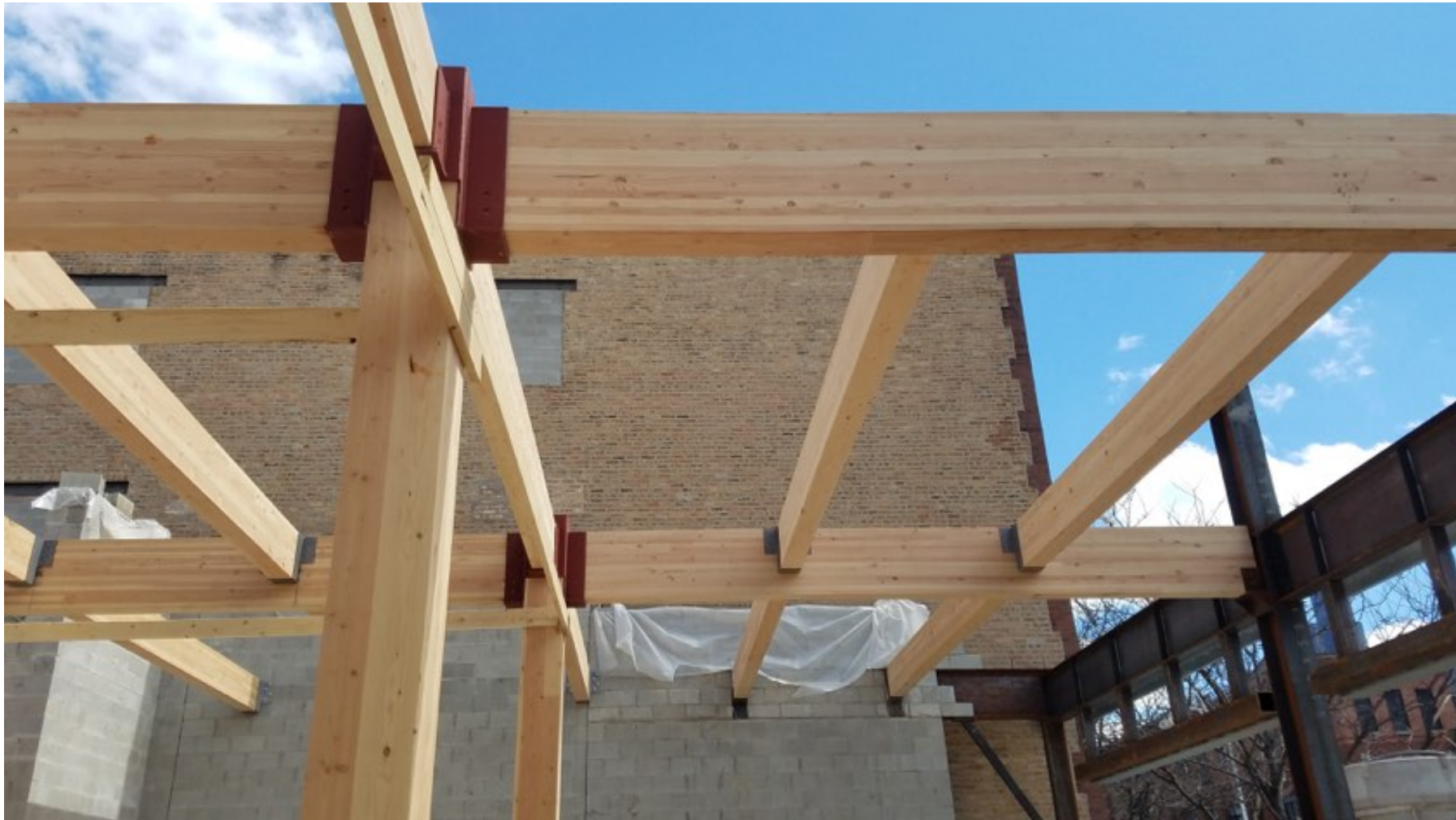
BEAM AND PURLIN CONNECTIONS
