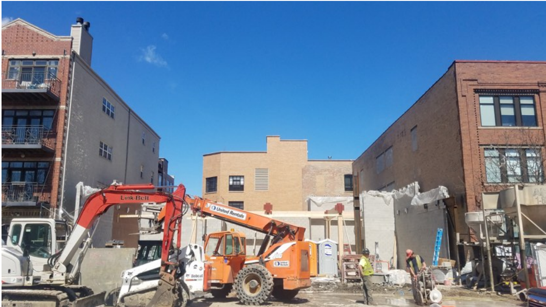
1ST FLOOR WALLS AND INITIAL TIMBER BEAMS BEING INSTALLED
