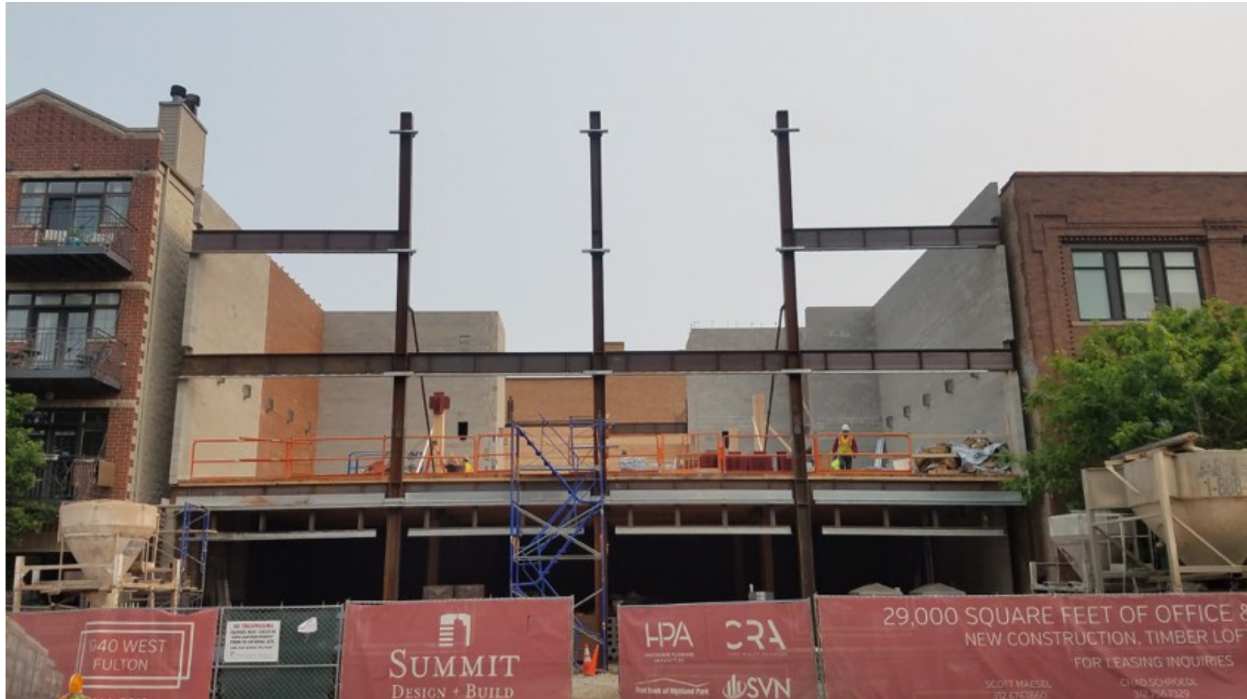
EXTERIOR WALL SUPPORT STEEL INSTALLATION
