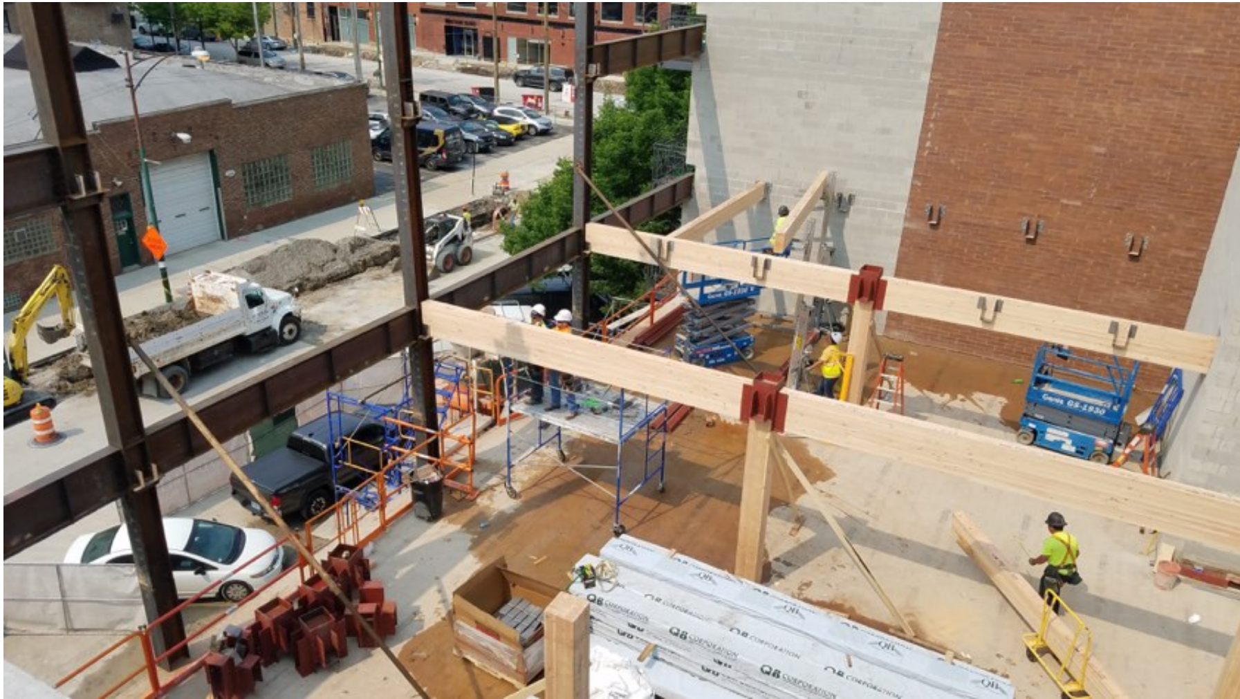
TIMBER FRAMING AT 2ND AND 3RD FLOOR
