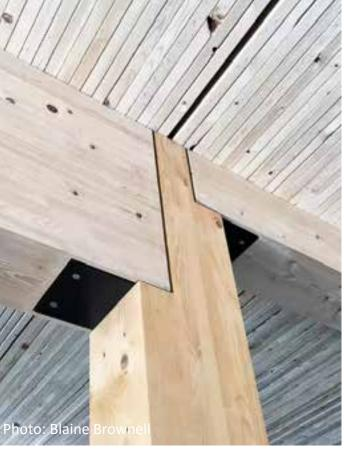
2017 Glulam Beam to Column Connection Fire Tests under standard ASTM E119 time-temperature exposure
