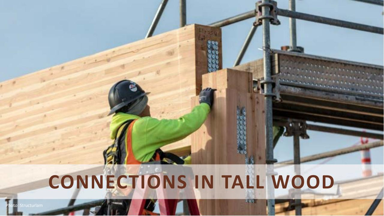
In Construction Types IV-A, IV-B & IV-C, building elements are required to be FRR as specified in IBC Tables 601 and 602. Connections between these building elements must be able to maintain FRR no less than that required of the connected
