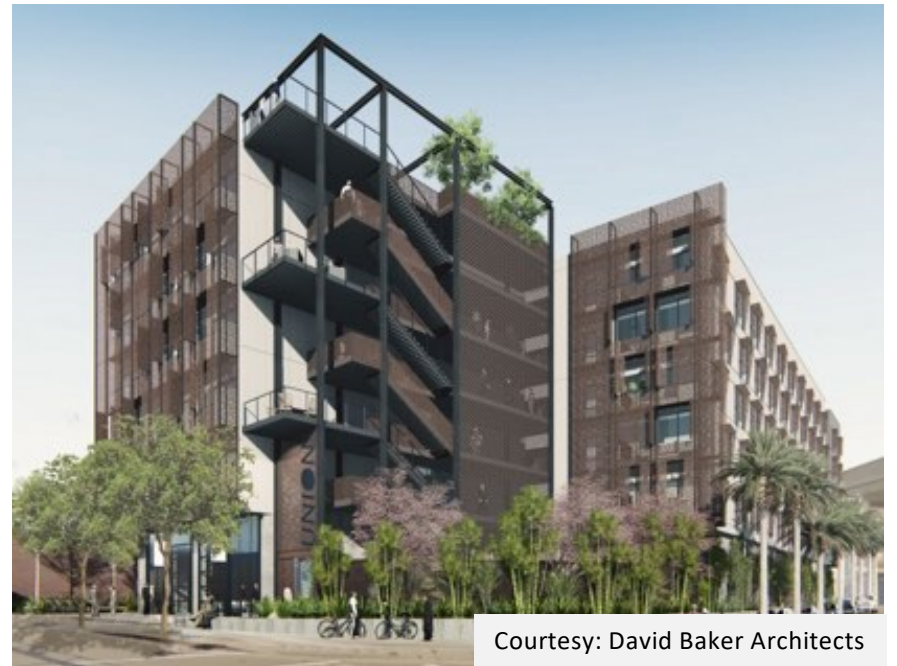
Courtesy: David Baker Architects
