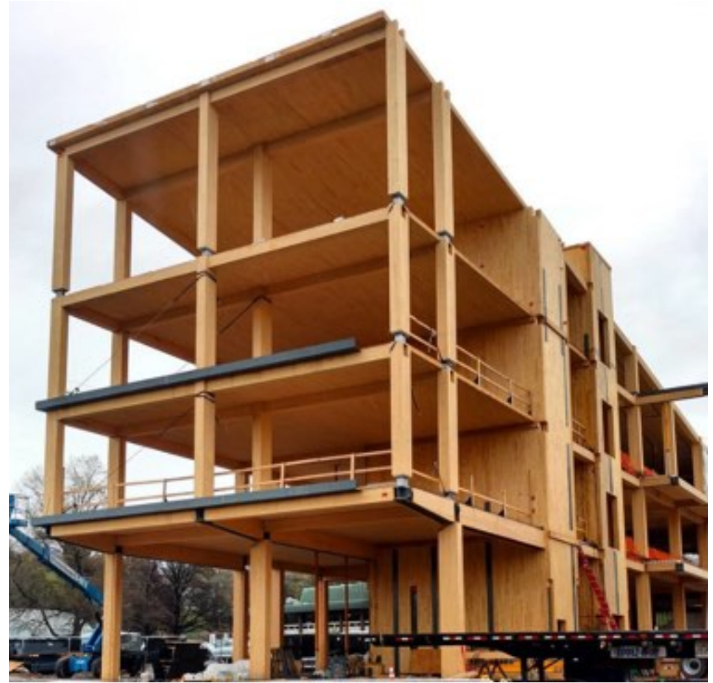
Mass timber mid-rise
