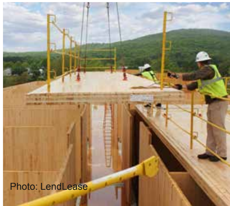
Cross-Laminated Timber (CLT) Solid sawn laminations
