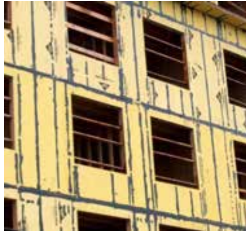
Sealed Gypsum Sheathing – Sealant Filler at Joints
