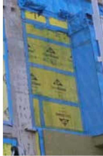
Sealed Sheathing – Membrane at Joints
