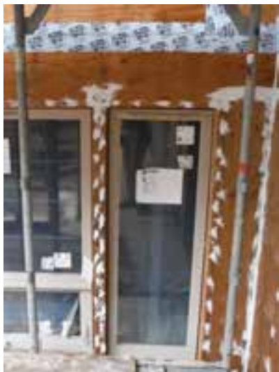
Sealed Plywood Sheathing – Sealant & Membrane at Joints
