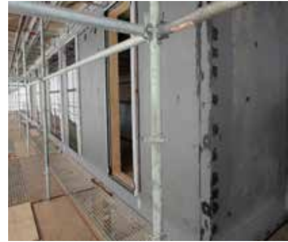
Liquid Applied – Silicone or hybrid sealants (STPE) and membrane
