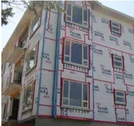
Loose Sheet Applied Membrane – Taped Joints & Strapping
