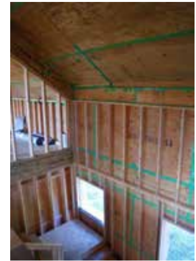
Plywood sheathing with taped joints (good tape)
