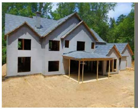
Integrated Air & Water Barrier System Applications
