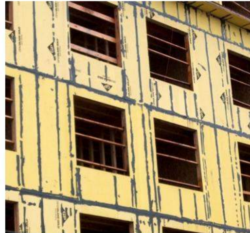
Sealed Gypsum Sheathing - Sealant Filler at Joints
