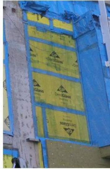
Sealed Sheathing - Membrane at Joints
