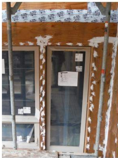
Sealed Plywood Sheathing - Sealant & Membrane at Joints
