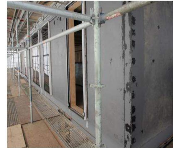
Liquid Applied - Silicone sealants and silicone membrane at Joints
