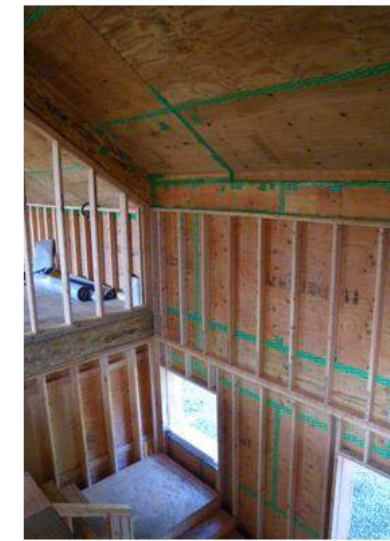
Plywood sheathing with taped joints (good tape)
