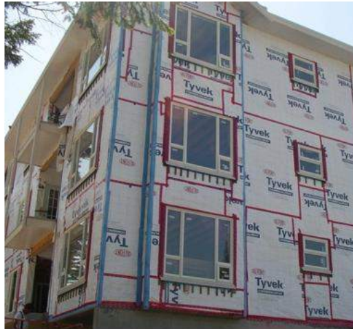
Loose Sheet Applied Membrane - Taped Joints & Strapping
