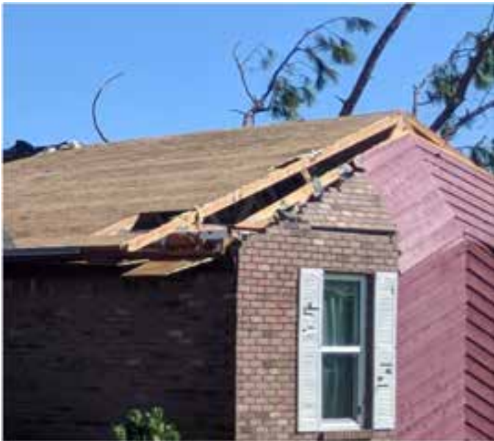
Gable-end Roof Damage
