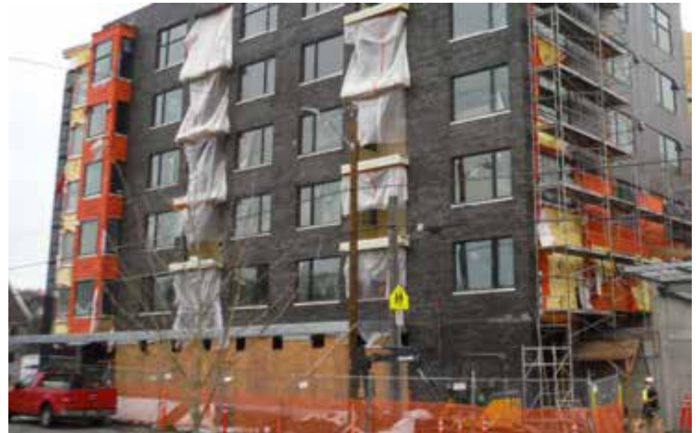
Fig. 3-2 Wood-Framed Wall with Anchored Masonry Veneer Example Project Application
