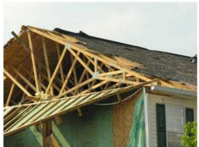
Gable-end Roof Damage
