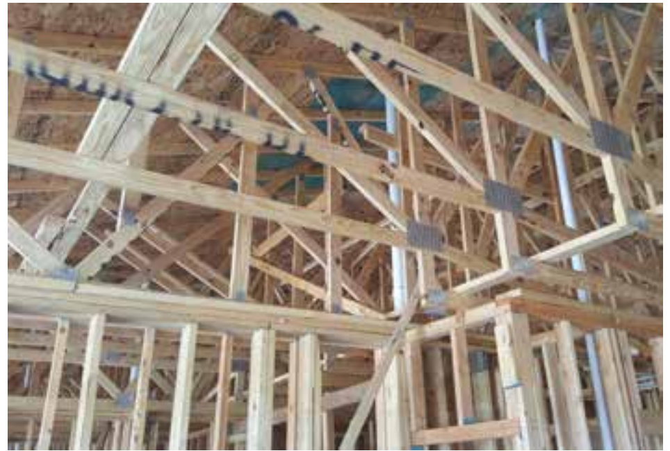
ROOF TRUSSES INSTALLED
