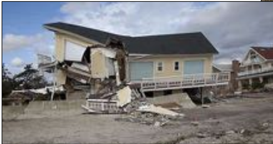
Possible Soft Story (Not enough shear walls across front)
