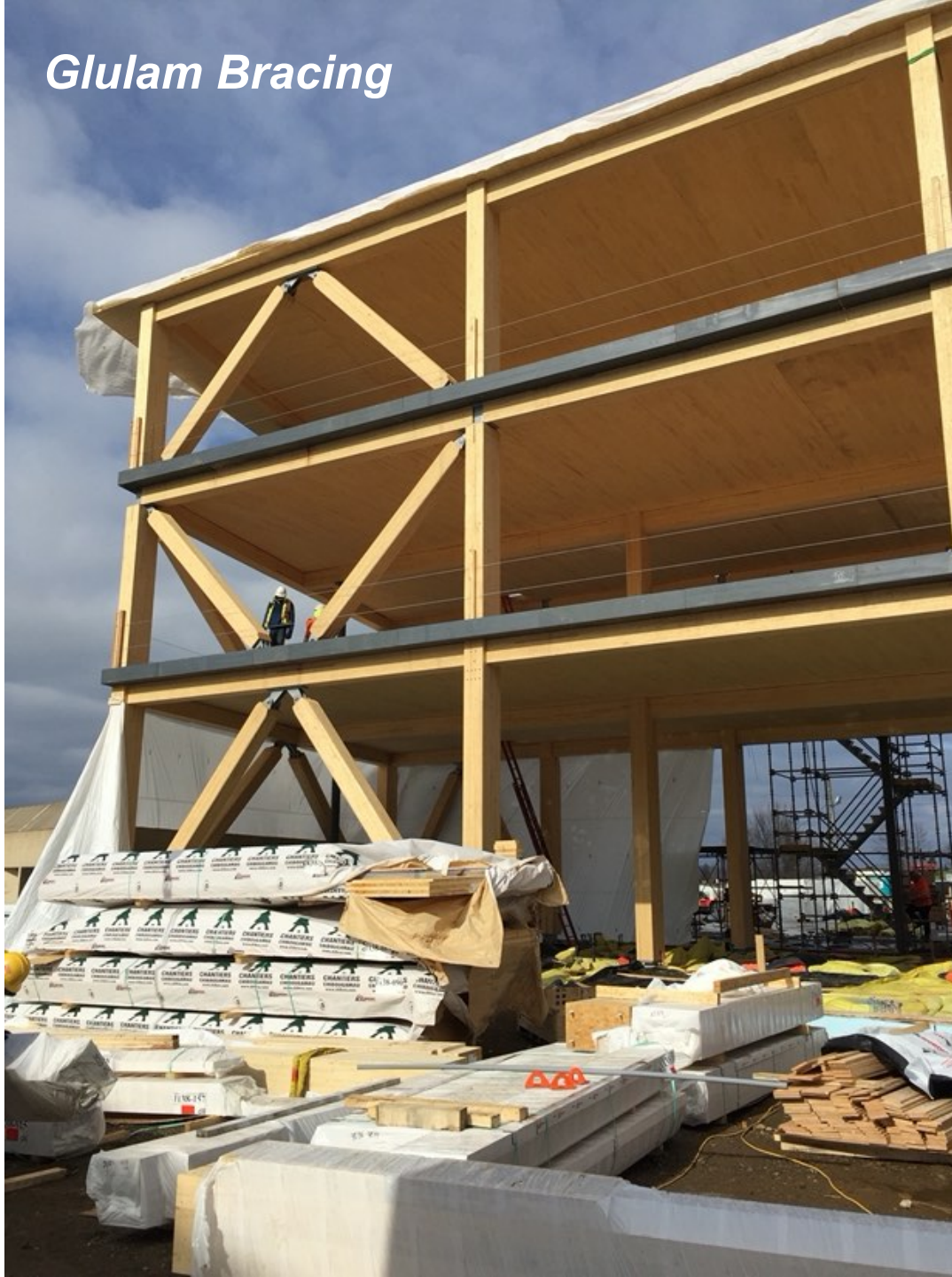
Lateral Cross Bracing
