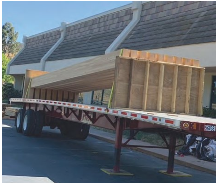
Skylight Component Pre-Assembled & Loaded
