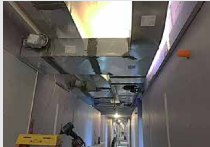
Ventilation Ducts appear to be well sealed with mastic.
