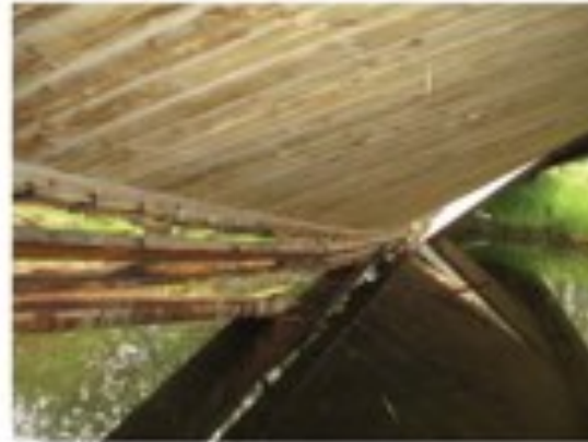
Cracked ledger and glulam
