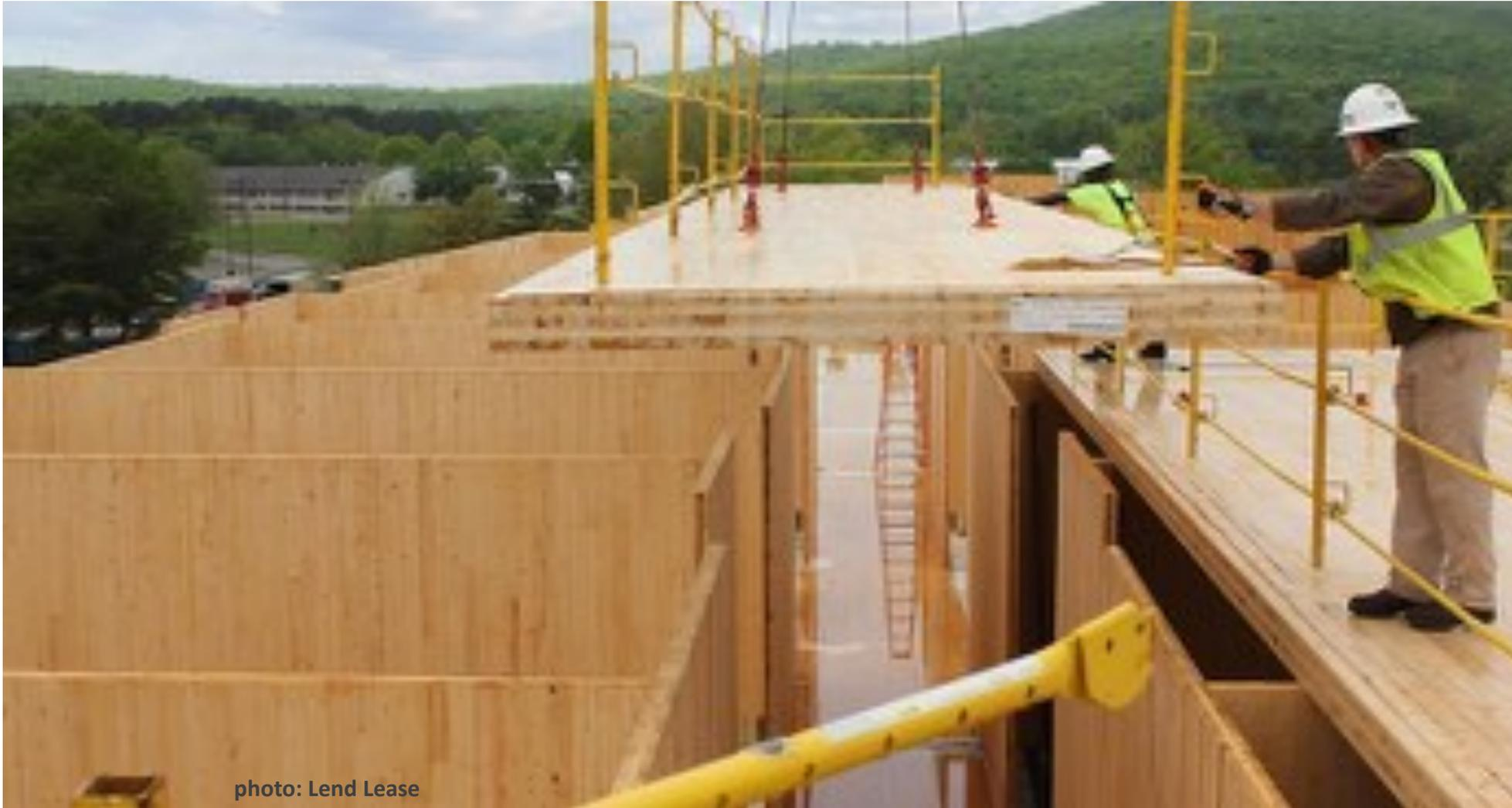
CLT Bearing Walls /Slabs
