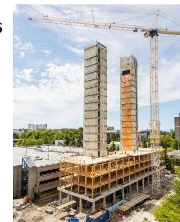
**Connections to concrete core**
