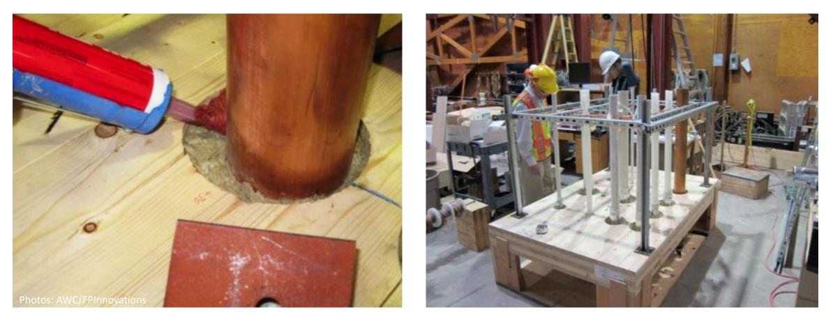
Most firestopping systems include combination of fire safing (eg. noncombustible materials such as mineral wool insulation) plus fire caulk
