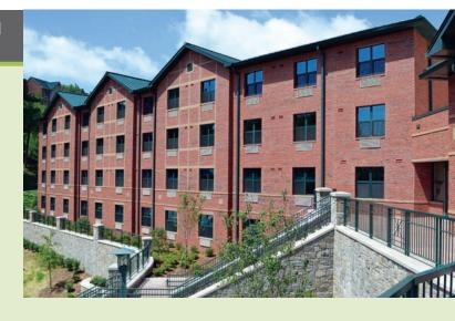
The bottom level of the four-story portion, where it was inset into the hillside, was traditionally framed on site, and three stories of modular units were then placed on top. The three-story portion of the project was entirely modular. All plumbing and drain lines were installed underneath the building before the modules were set. In fact, everything had to be ready at the site, because the modules took only 30 days to lift into place.
